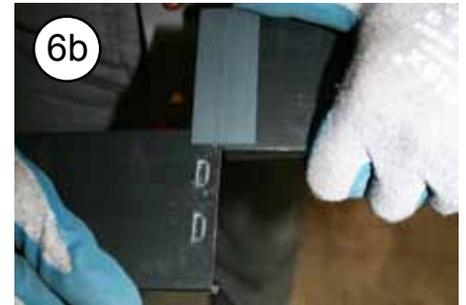
Place the clamping ring around the top edge of the cover insulation. The ring is closed with a connection strip (6a, 6b), similar to the connection strips for the insulation mats.
