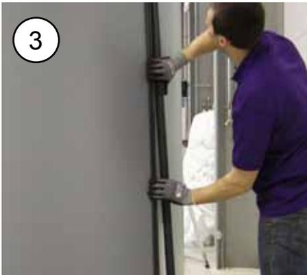
After joining the insulation mats along the entire circumference (3), lock the end pieces together with the aluminium closure strip patented by ECOTHERM.
