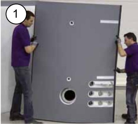
Remove the insulation mats from the packaging and position them around the connections on the storage tank.
