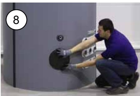
As a final step, fit the flange insulation: First insert the fibre fleece disk. Then push the cap over the insulation (8a).
