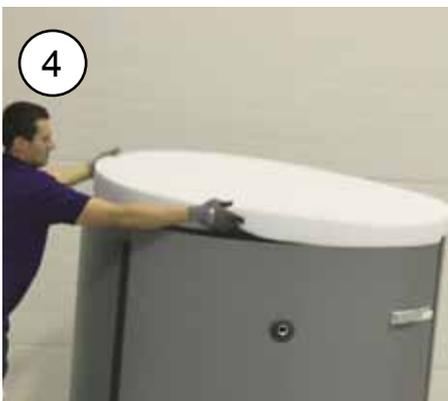
Now install the cover insulation: First lay the fibre fleece disk onto the cylinder (4), then position the polypropylene cover on top (5).
