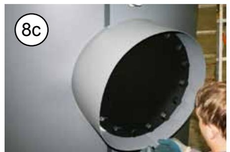
For larger flanges that DN 200 there exists a large flange insulation, which can be easily installed according to the steps 8b to 8d.
